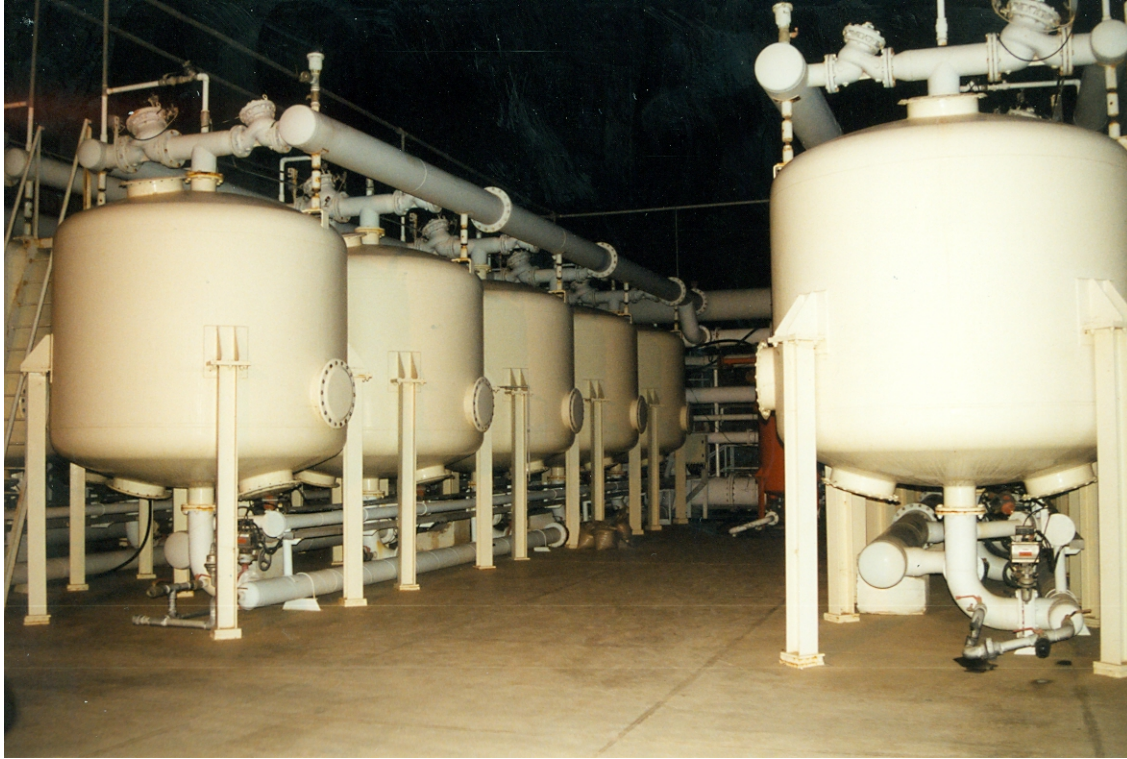
Figure 3. The sizing of the filtration system can be accomplished by either using filtration units with greater area of filtration or through usage of multiple filtration units in parallel (bank of filters). For this filtration system for microirrigation in the Canary Islands using wastewater, both techniques for sizing were employed. For scale, these sand media tanks are approximately 12 feet in height. (Photo courtesy of Freddie Lamm, Kansas State University)
