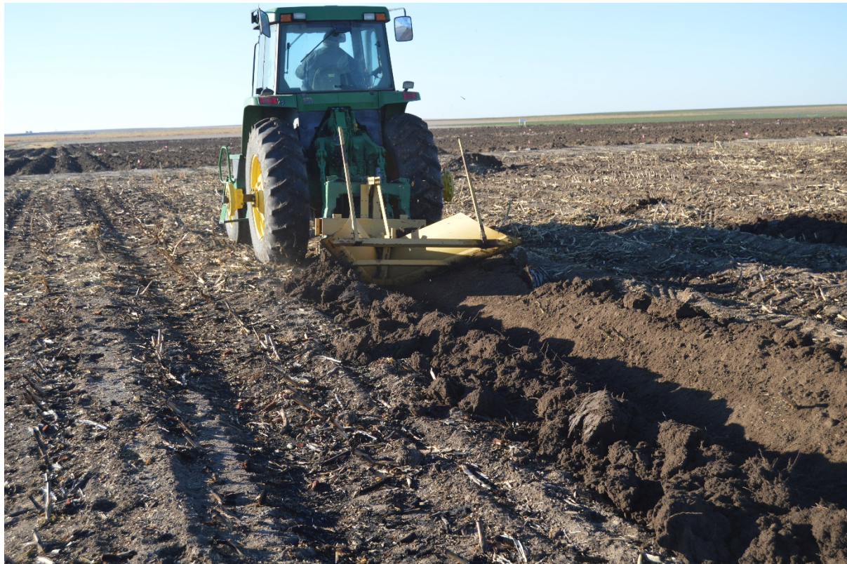
Figure 4. Excavating the overburden over driplines selected for laboratory performance measurements.
