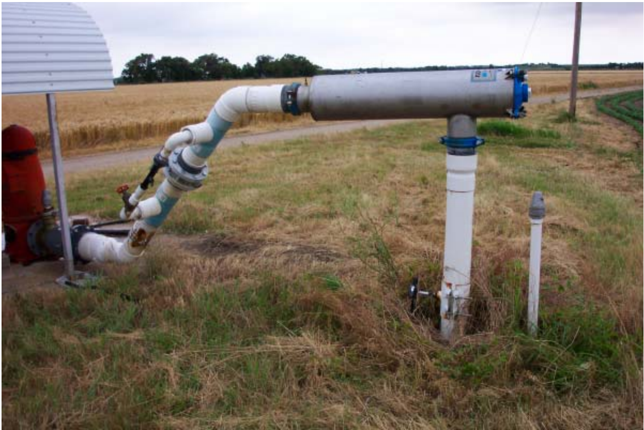
Figure 3a: Original pumping plant and filtration configuration of the case study SDI system.
