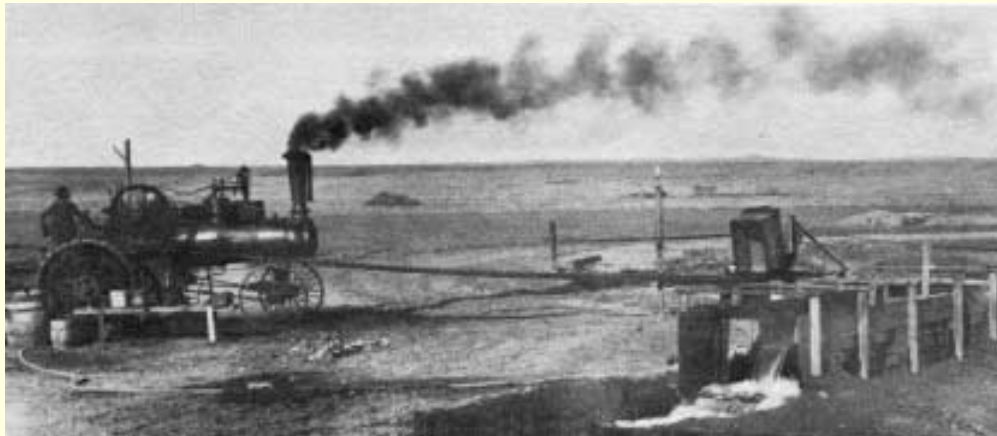
Pumping water for irrigation from a well near Big Creek in Hays vicinity, Ellis County, early 1900s. A centrifugal pump operated by a steam engine, using a thresher belt.
