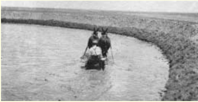
Puddling reservoir, Garden City Branch Station, 1914. Puddling was necessary to reduce water loss by seepage.
