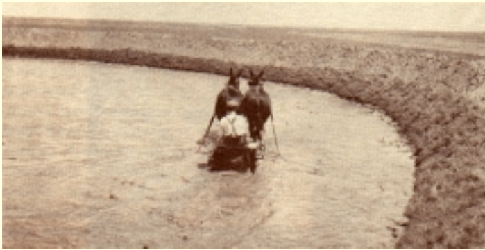
Puddling reservoir, Garden City Branch Station, 1914. Puddling was necessary to reduce water loss by seepage.
