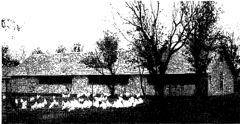
FIG. 3.—This 20- by 70-foot house consists of three rooms, each 20 feet square, and a service room 10 by 20 feet on the left. This is a desirable 300-hen unit where poultry is an important department on the farm.
