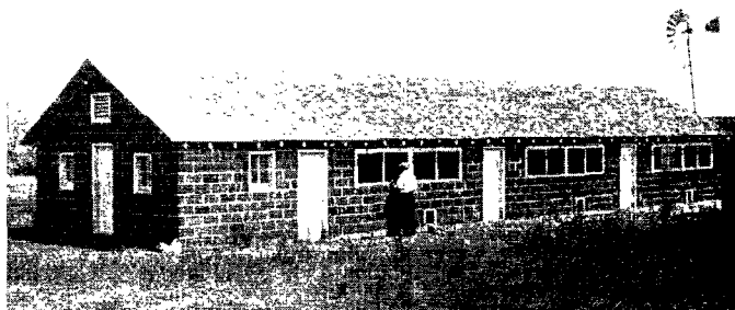
FIG. 6.—A 20- by 70-foot glazed-tile house for 300 hens. (Farm of E. J. Mall, Clay Center, Kan.)
