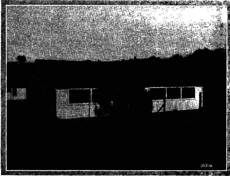
Fig. 3.—Front view of the Kansas 20- by 40-foot open front, gable roof, straw loft poultry house.
