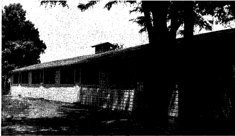
FIG. 15.—The house shown in figure 1 after it was remodeled in 1926 for Experiments IX, X, and XI. A straw loft was installed and the large openings in front admitted direct sunshine and improved the ventilation.
