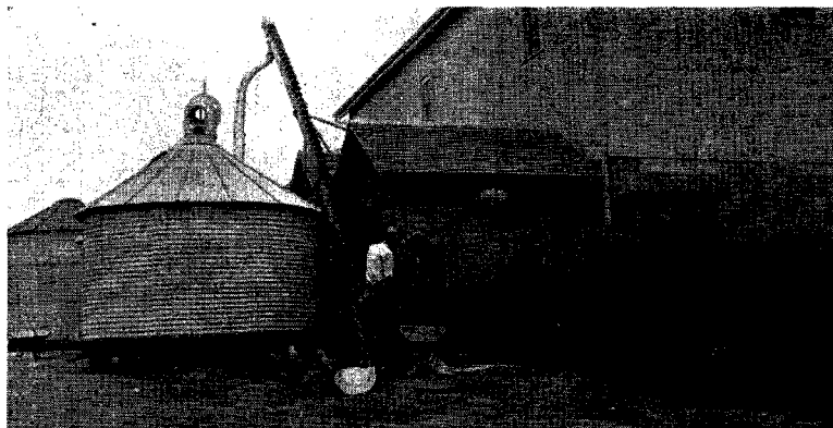
FIG. 9.—Filling the bins with damp wheat by use of the John Deere tubular grain elevator, summer, 1929.
