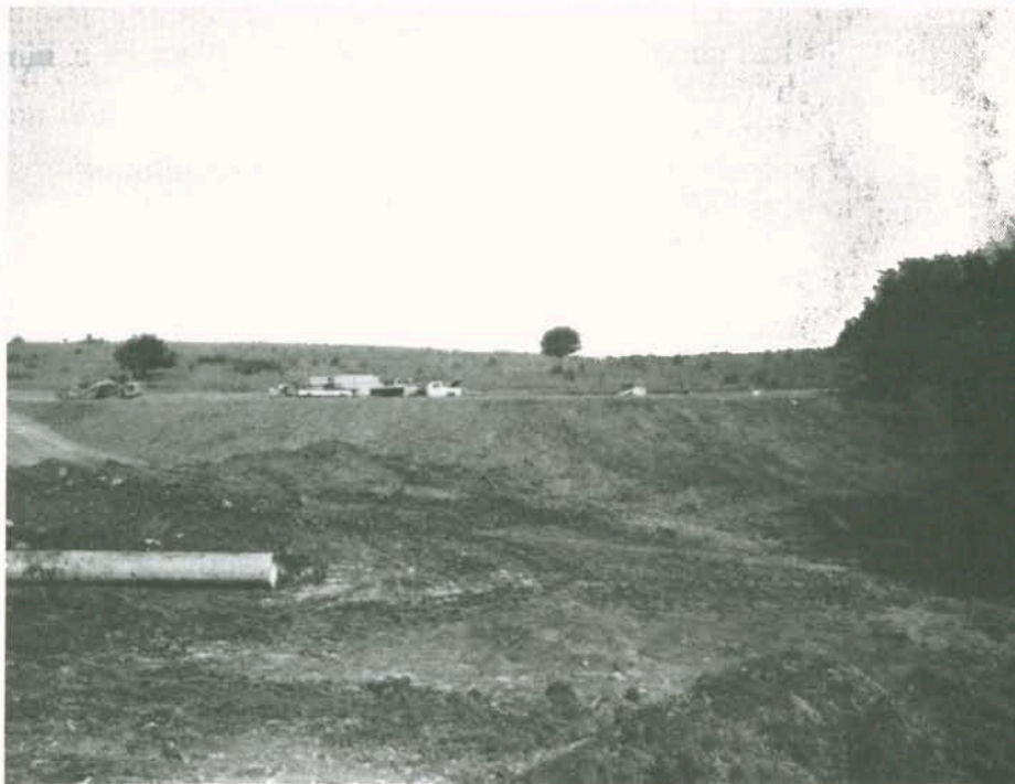
Site Preparation of the New KSU Segregated, Early-Weaning Facility.
