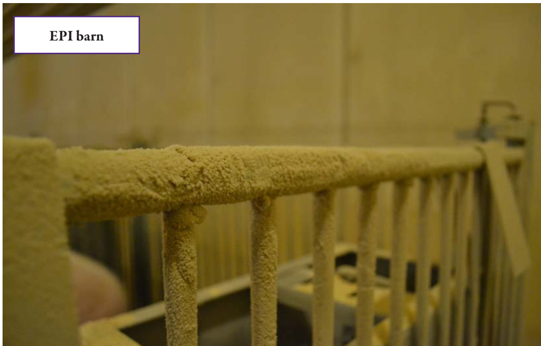
Figure 1. Dust accumulation on pen railing in experimental barns.
