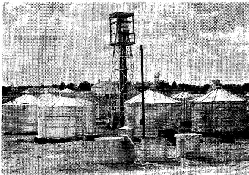
Fig. 47.—Grain storage bins were used to study the effect of ventilation upon the removal of moisture, cooling, and prevention of damage in stored wheat.
