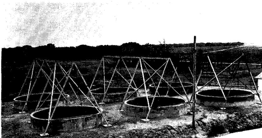
Fig. 20.—Battery of pit silos 19 feet in diameter and 35 feet deep built with the assistance of the Works Progress Administration. This construction “furnished much labor during 1935 and 1936.”
