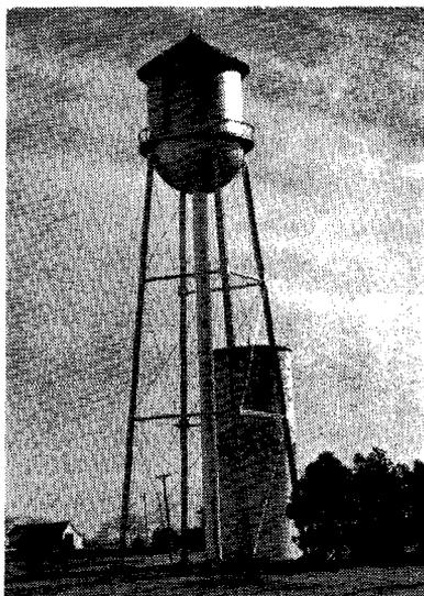
Fig. 21.—New water tank, with old concrete water tank in background. This 50,000-gallon tank was purchased in August, 1938, and erected during the winter months.
