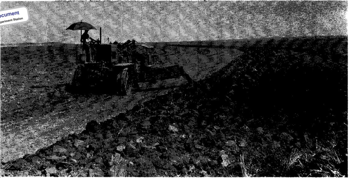
Fig. 71.—An elevating grader was used to construct some 10 miles of terraces to conserve water and to control soil erosion on the cultivated land of the Station.
