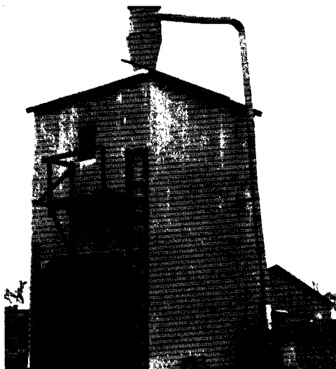
FIG. 29—A convenient method of grinding and feeding sorghum roughages. The feed is blown from the hammer mill into an elevated bin. Trucks or wagons are loaded from a trap door in the sheltered area where the wind does not interfere and waste feed.
