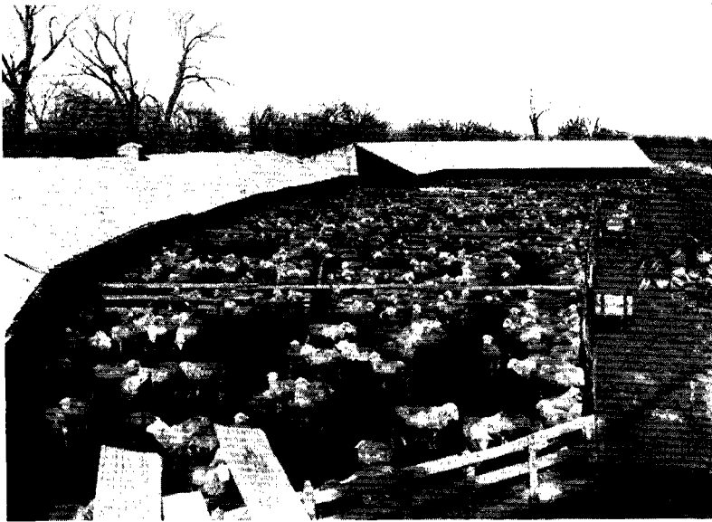
FIG. 7.—An open-front shed affording protection overhead and also from north and west winds. This shed, which has capacity for 3,500 to 4,000 lambs, is of an inexpensive yet adequate type.
