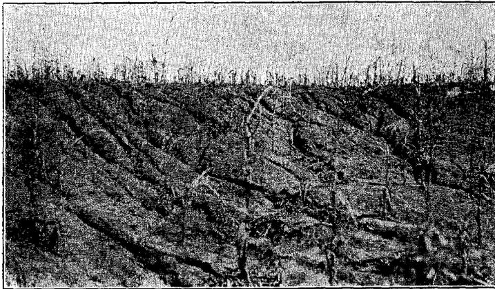
Fig. 1.—Severe erosion caused by listing up and down a slope. Such fields should be seeded permanently to grass
