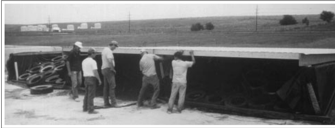
A cover or roof on a horizontal silo will greatly reduce dry matter losses and preserve silage quality.
