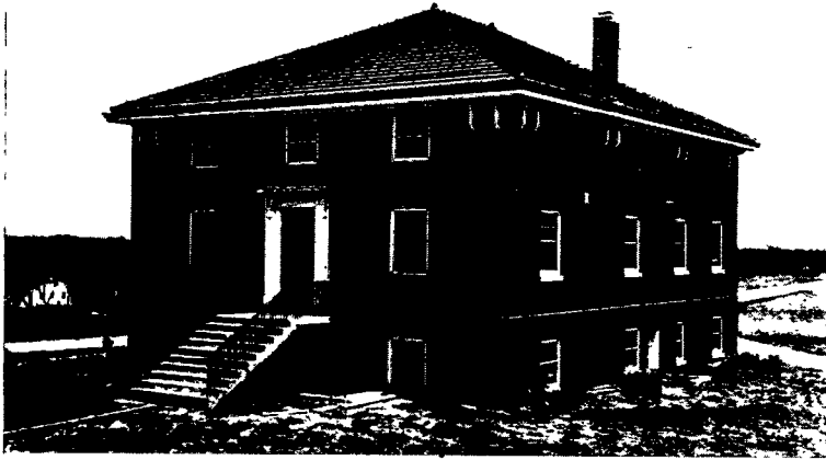
FIG. 2.—New crops-and-soils laboratory building at the Fort, Hays Branch Experiment Station, Hays, Kan.
