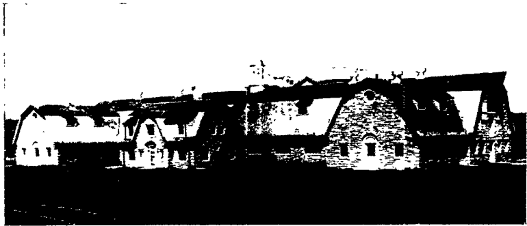
FIG. 1.—New dairy barn and dairy experimental laboratory.
