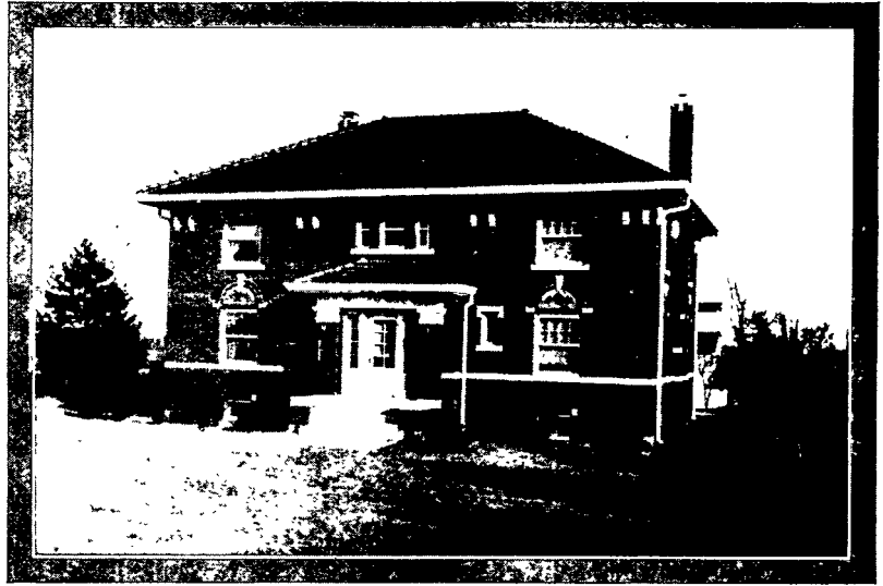
FIG. 2.—The new residence of the superintendent, Fort Hays Branch Experiment Station.
