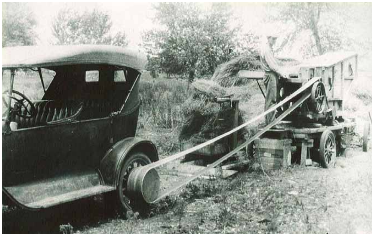
Threshing flax plots at the Southeast Kansas Experiment Field with unique power source developed by Superintendent Floyd Davidson, circa 1923.
